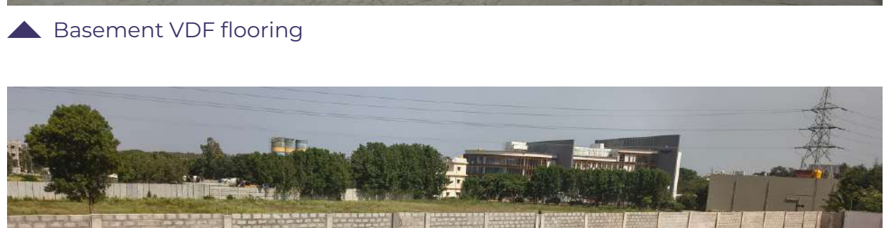
▲ East side compound wall work
