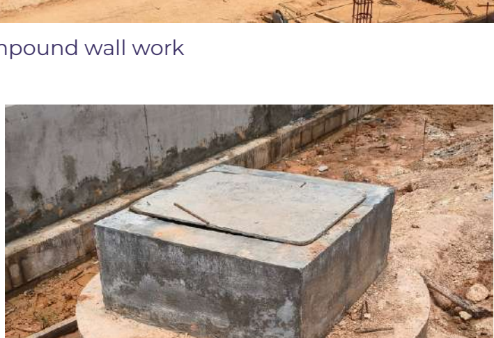
▲ Recharge percolation pit work
