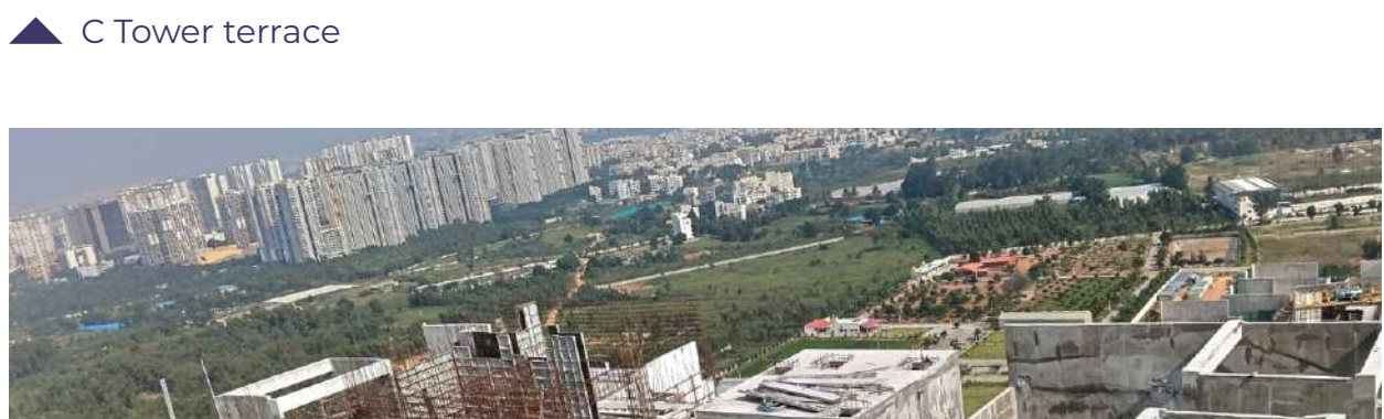
▲ Terrace parapet wall work in progress
