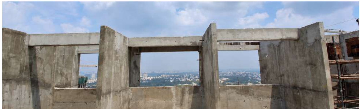
▲ Internal walls putty work
