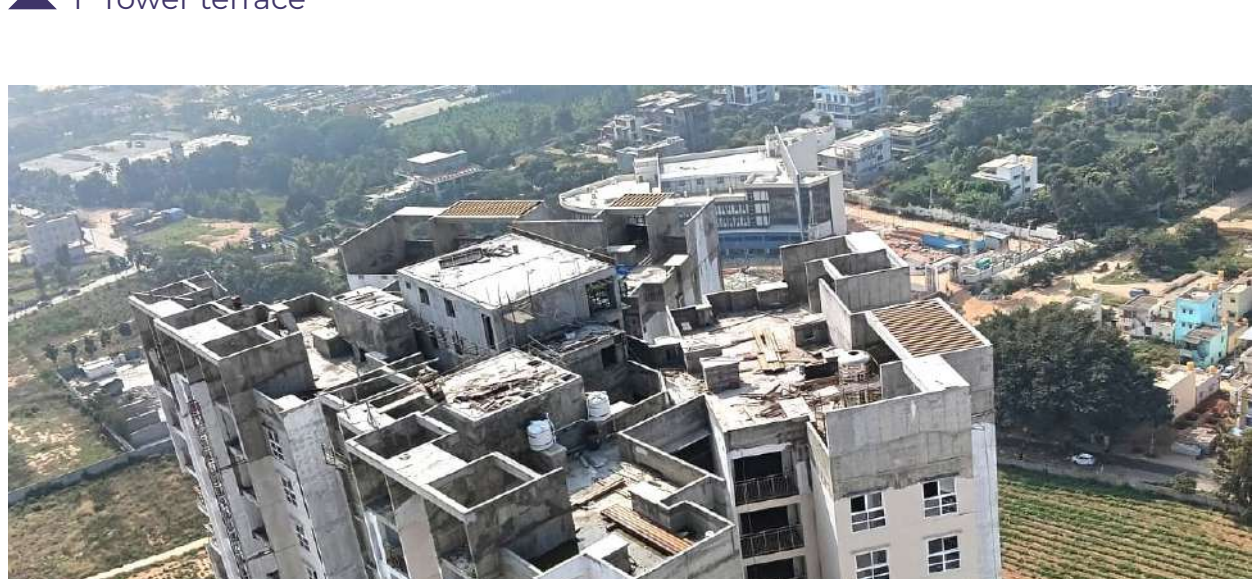
▲ Terrace pergola work in progress
