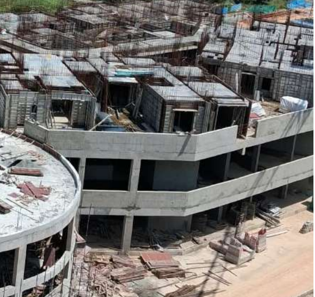
▲ Stormwater drain work in progress
