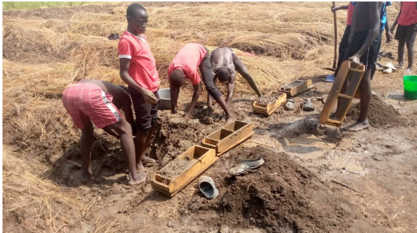
AFSS students making bricks to be used for the security fence.
