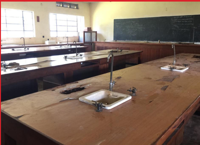
50-year-old SHS Science Lab before renovation.
