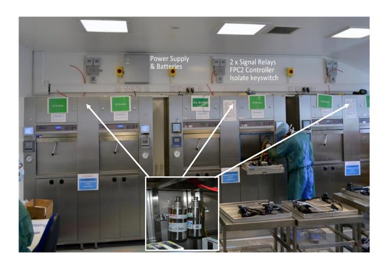
The proposed fire detection and automatic suppression system met client requirements and incorporated fire engineering basics, such as battery backed / monitored power supply, fault monitored circuitry and remote signalling to various ancillary plant.
