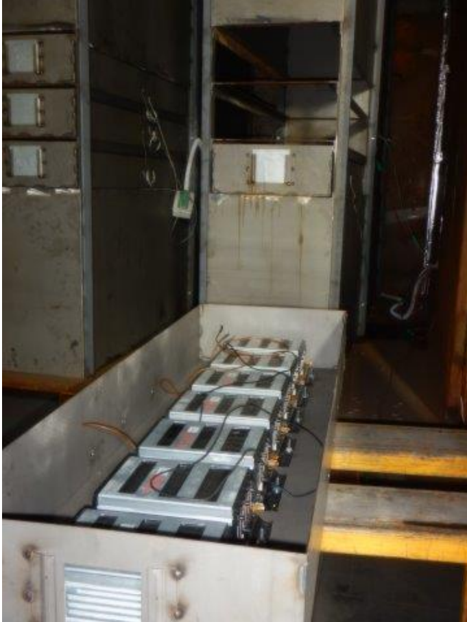
Sample: 2024407 - Picture #7 Positioning the battery housing inside the rack
