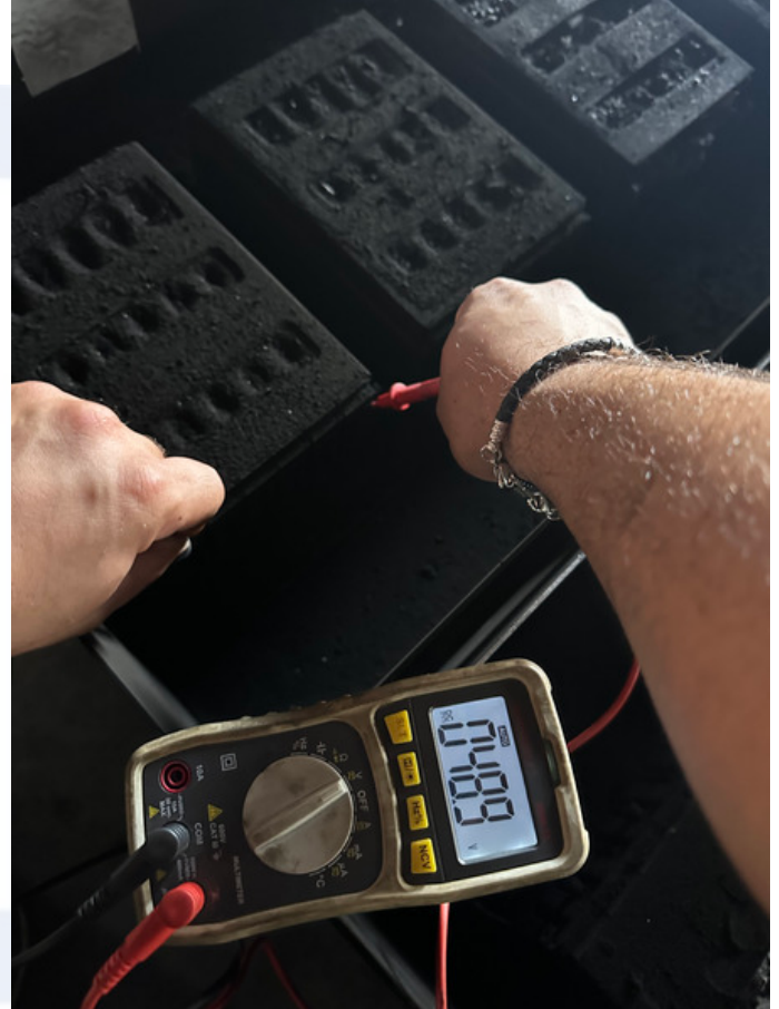
Sample: 2024408 - Picture #19 Surrounding modules still working after the test
