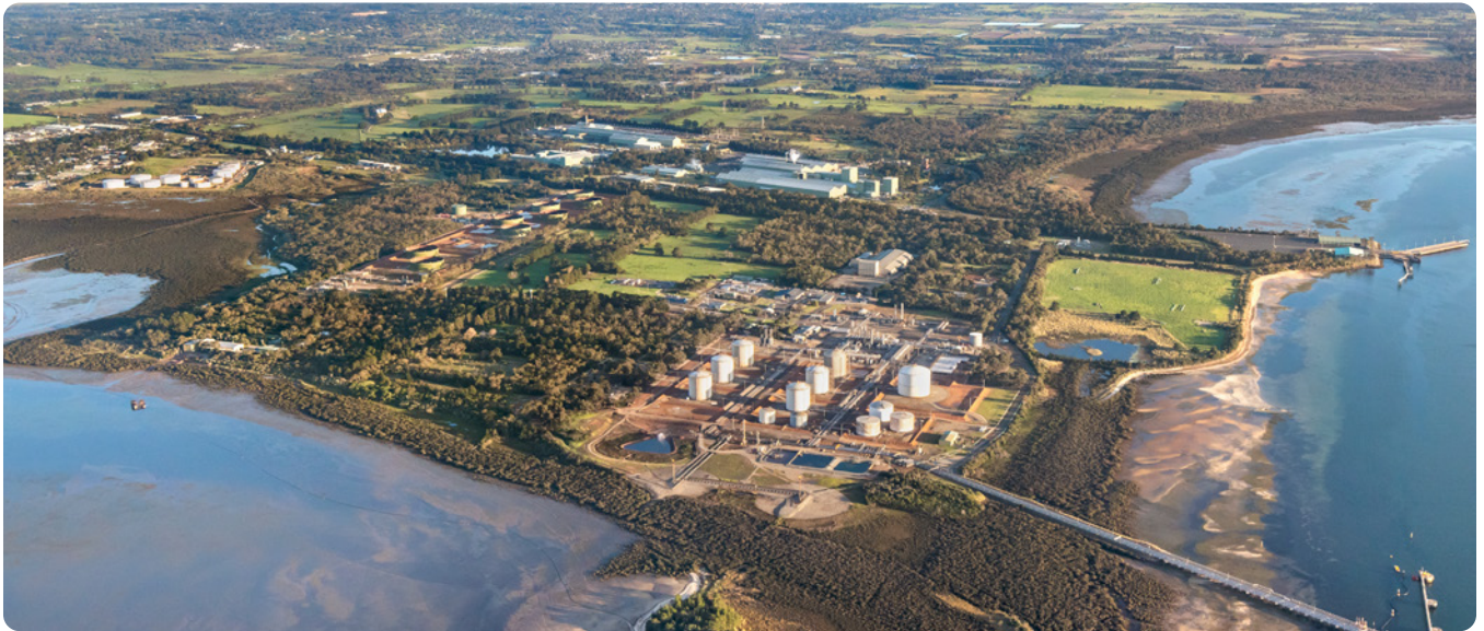
Image: Aerial of the Old Tyabb Reclamation Area and surrounding industrial precinct.
