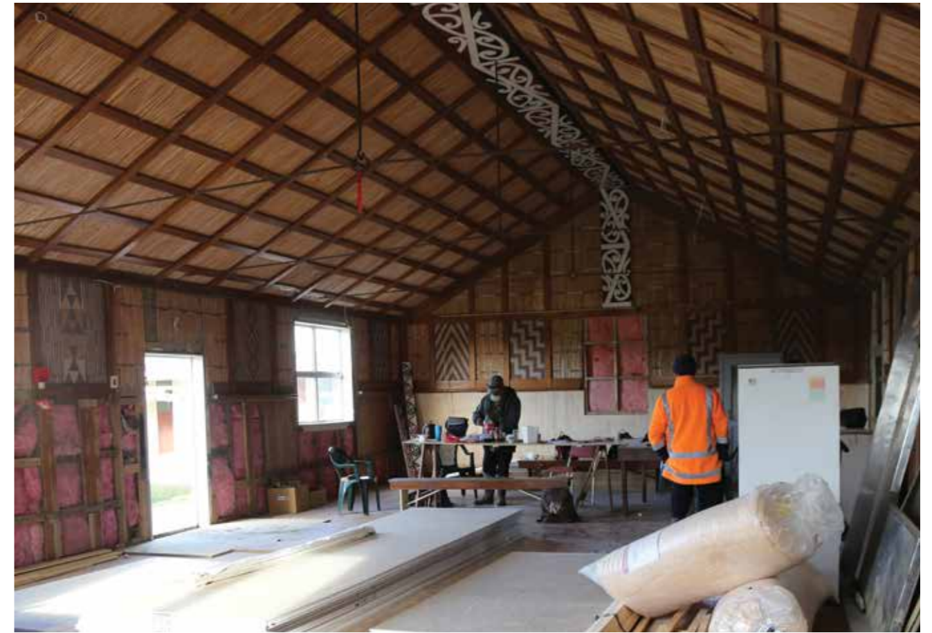
Above Renovations to wharekai at Tikapa Marae.
