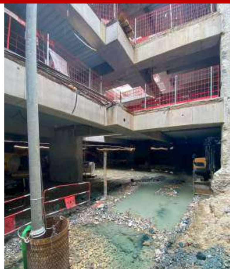
A ground water at -3 m
