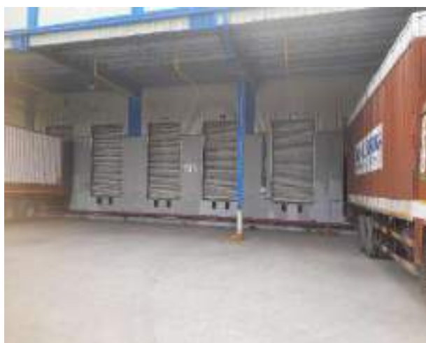
Dock Yard – Loading Point
