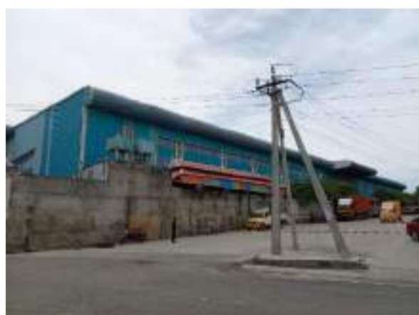
View of Subject Asset Compound Wall
