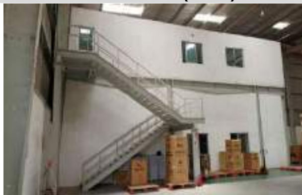
Internal View of Subject Asset
