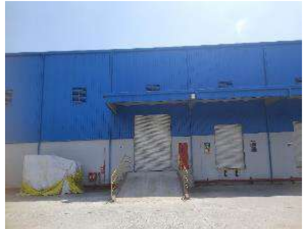
External View of Block
