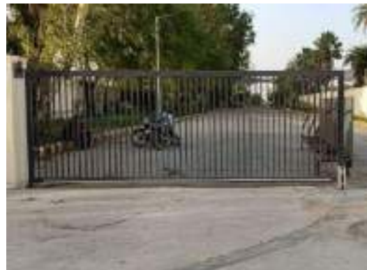
Entrance of Subject Property
