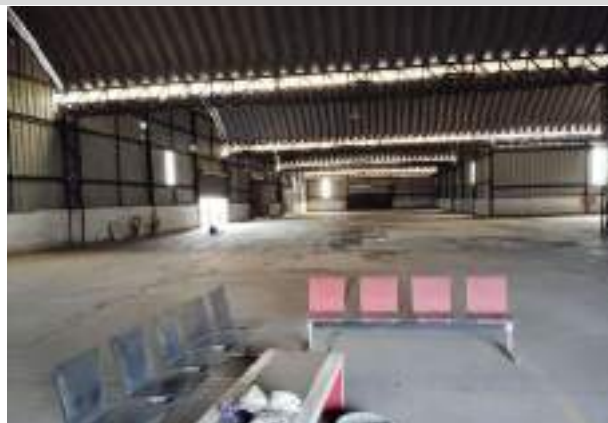
External View of Block
