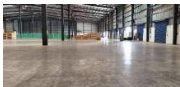
Internal view of Subject Property
