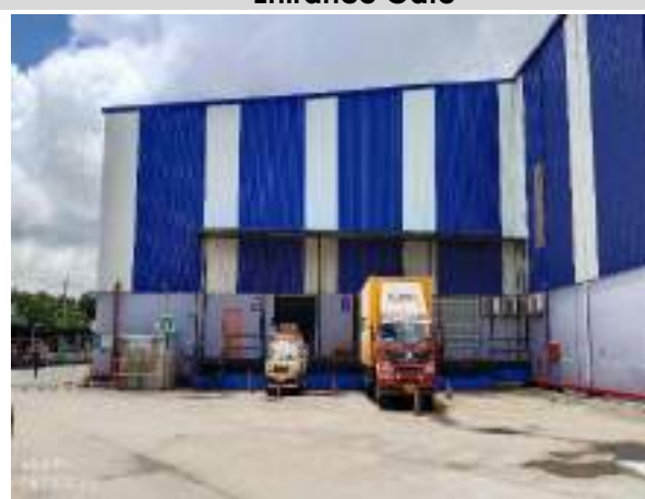
View of Loading Point
