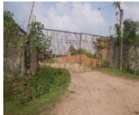
Subject Asset – Entrance Gate
