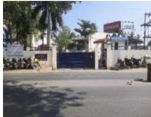
Subject Asset Entrance Gate
