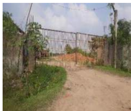
Subject Asset – Entrance Gate
