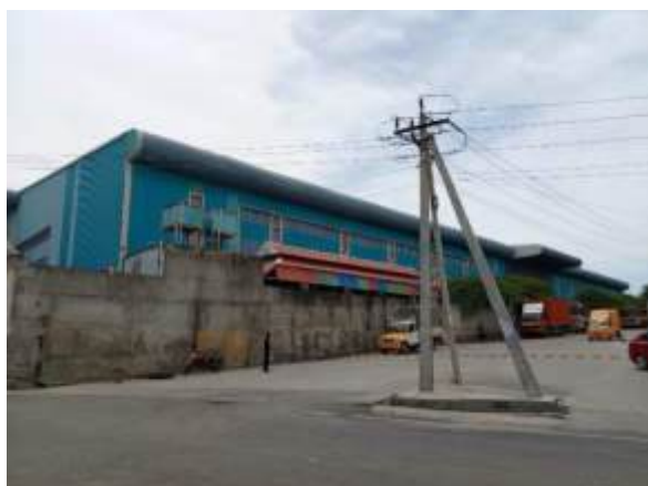
11) View of Subject Asset Compound Wall
