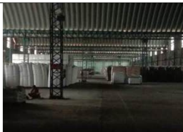
8A) View of Subject Asset
