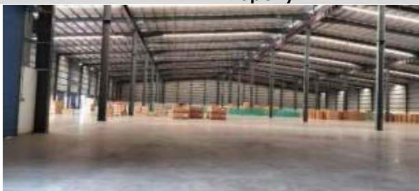
7) Internal View of Subject Property
