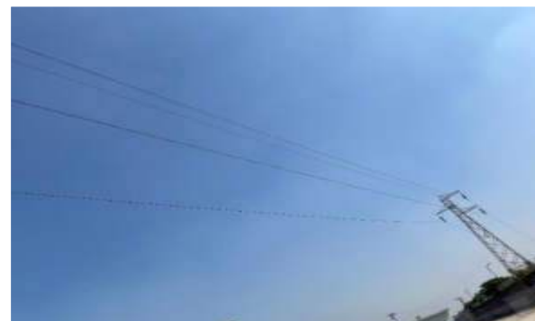
9) View of high-tension line crossing at site
