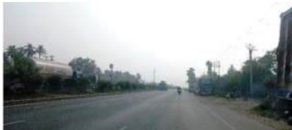
1) Access Road (NH16)
