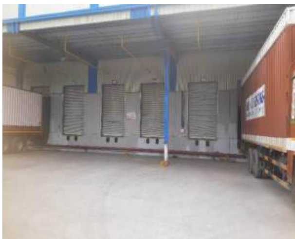
24) Dock Yard – Loading Point
