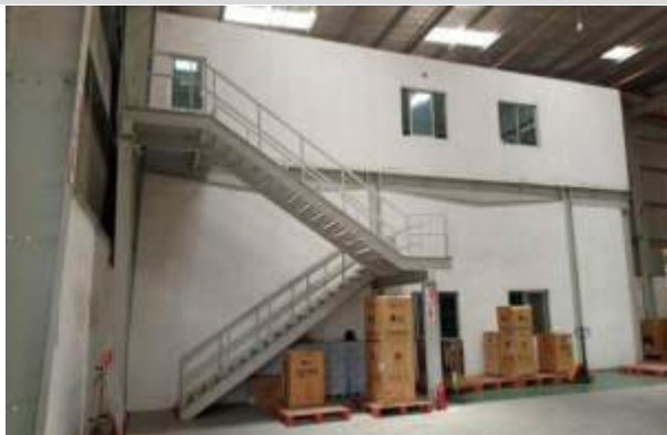
14) Internal View of Subject Asset
