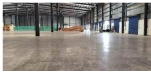
6) Internal view of Subject Property
