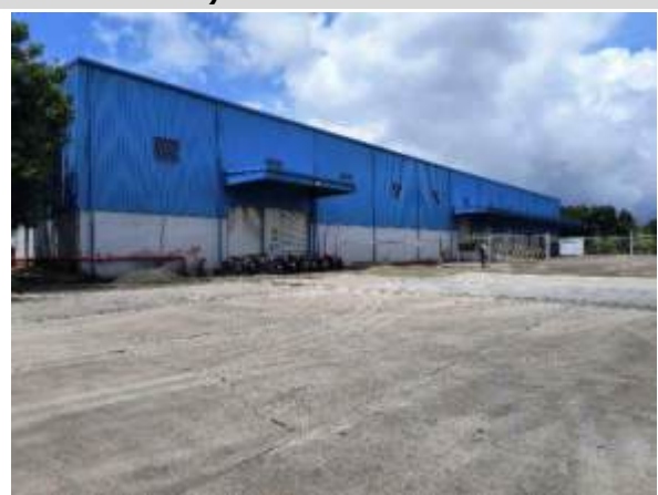
44) External View of Block
