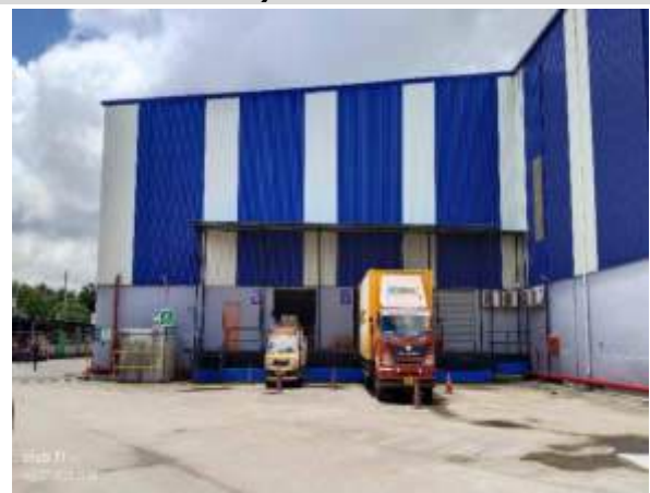
84) View of Loading Point
