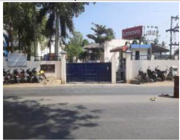
74) Subject Asset Entrance Gate
