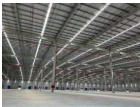
5A) Internal view
