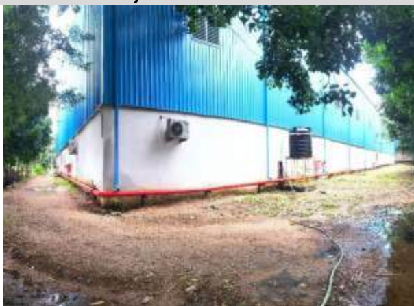
43) External View of Block
