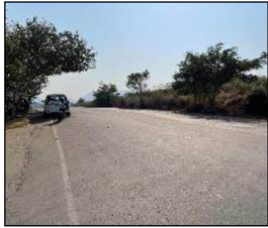
137) Access Road towards Chirner
