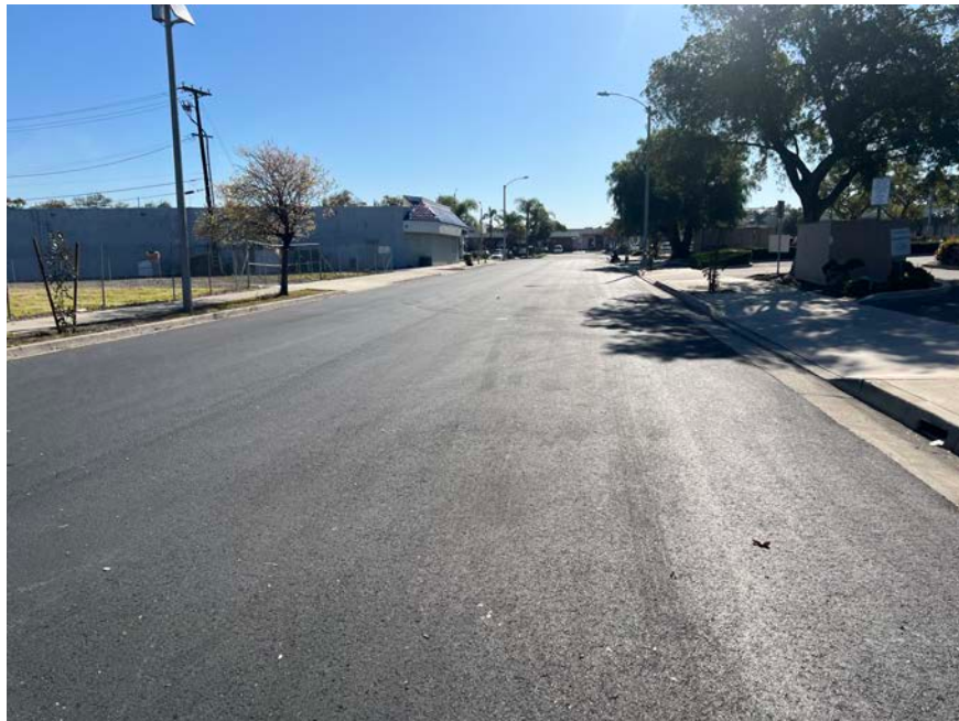
Looking to the East on 5 th Street
