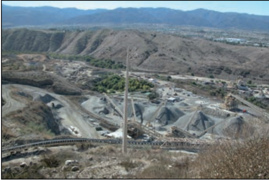
Figure 14: Material Sorting and Stockpiling
