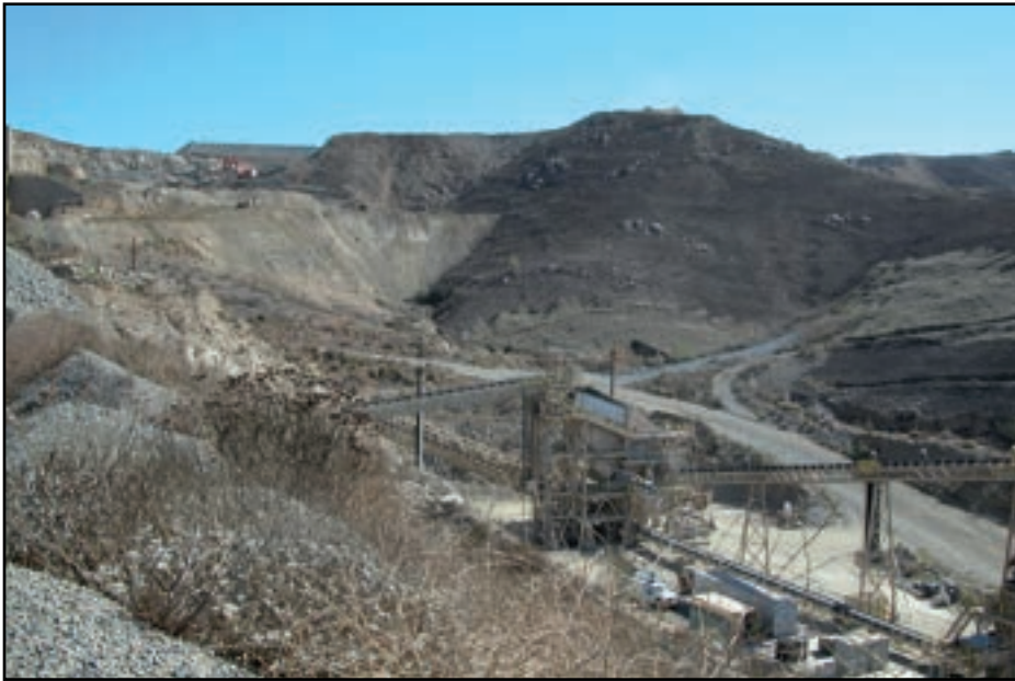
Figure 13: Material Processing and Conveyor Facilities
