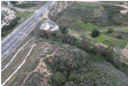
(7) Near center east edge of the Project Area facing south. Manufactured slopes and basin at the eastern end of Drainage 3.
