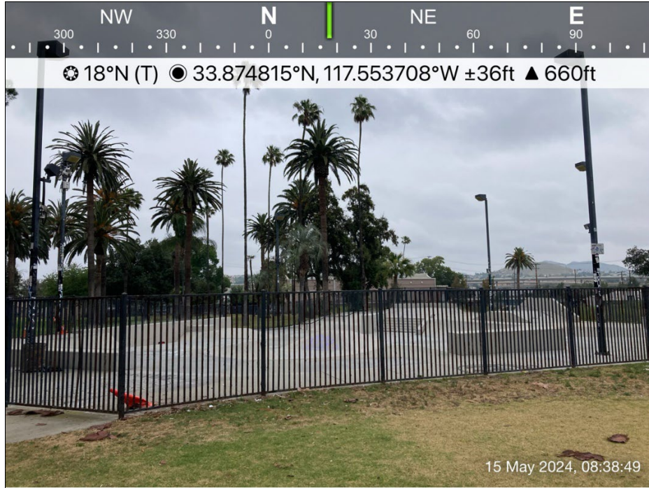
Photo 3. View of the Skate Park in the Southeastern Portion of the Project Site
