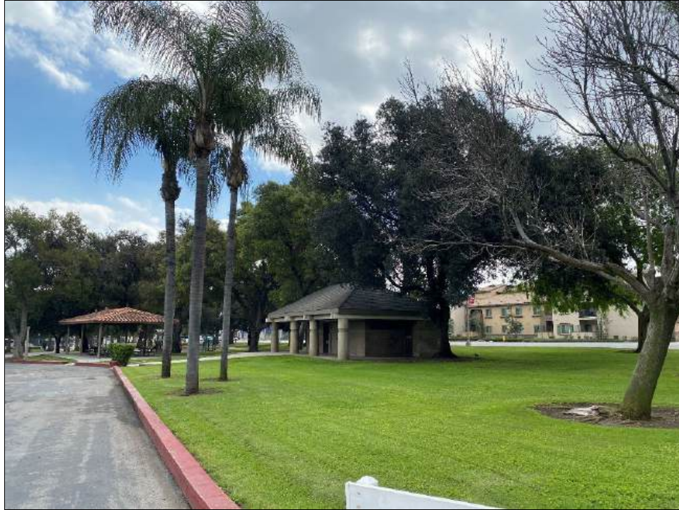
Figure 15. Circa 1990s Bathrooms and Picnic Shelter in the Southern Portion of City Park (view east; April 4, 2024).
