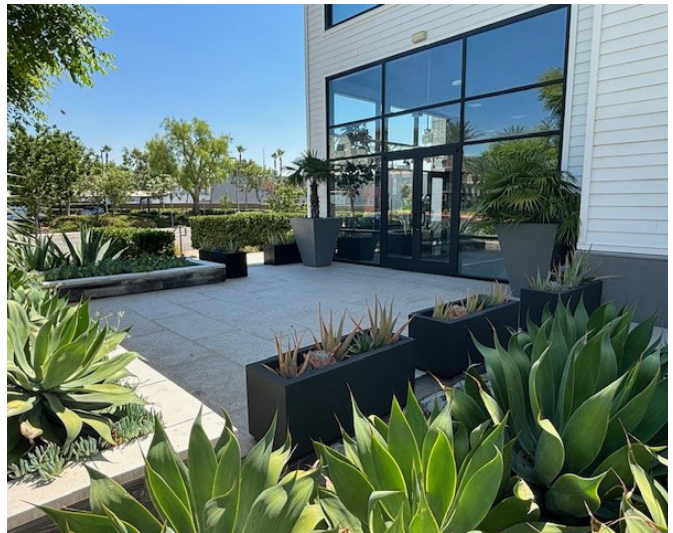
Landscape treatment complements building
