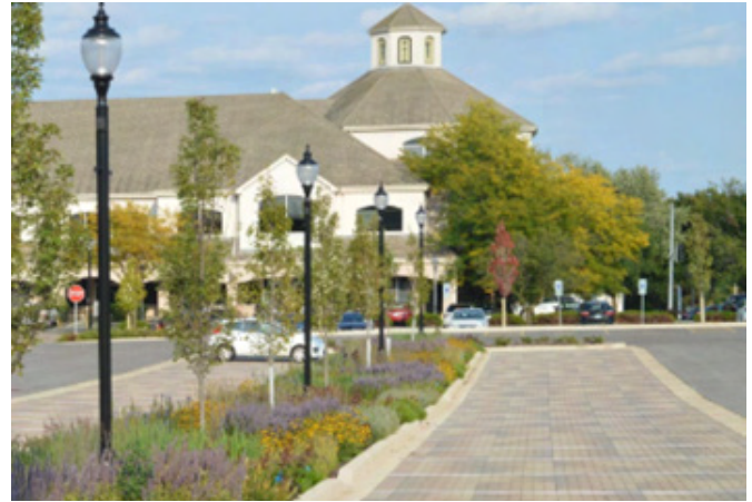
Porous paving in parking lot
