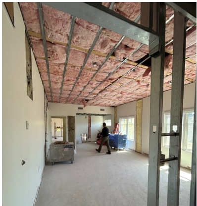
Construction sign and room under construction.
