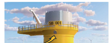
Skybox after installation
