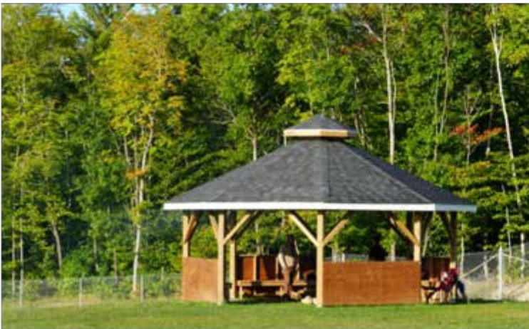
New Arbour constructed at Biidaaban Summer 2025
