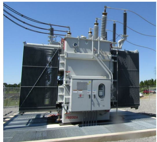
Figure 5. GSU Transformer with Secondary Containment to Capture any Leaked Oil
