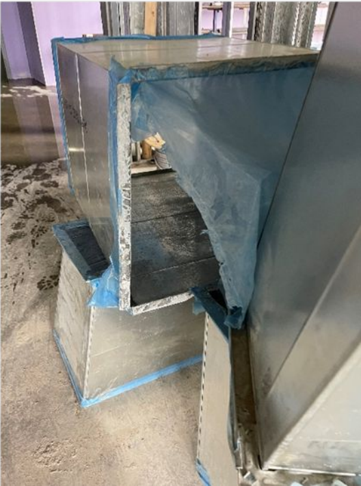
Protection of Ductwork
