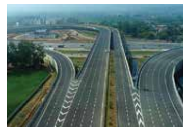
Nagpur - Goa Expressway*
