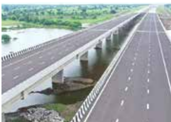
Mumbai - Nagpur Expressway*
