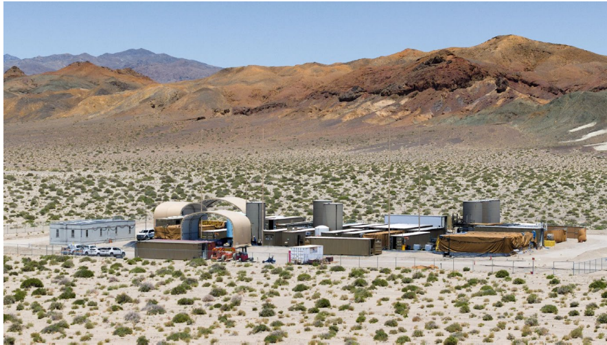
Nevada demonstration plant produced LCE on-site from sub-surface brine
