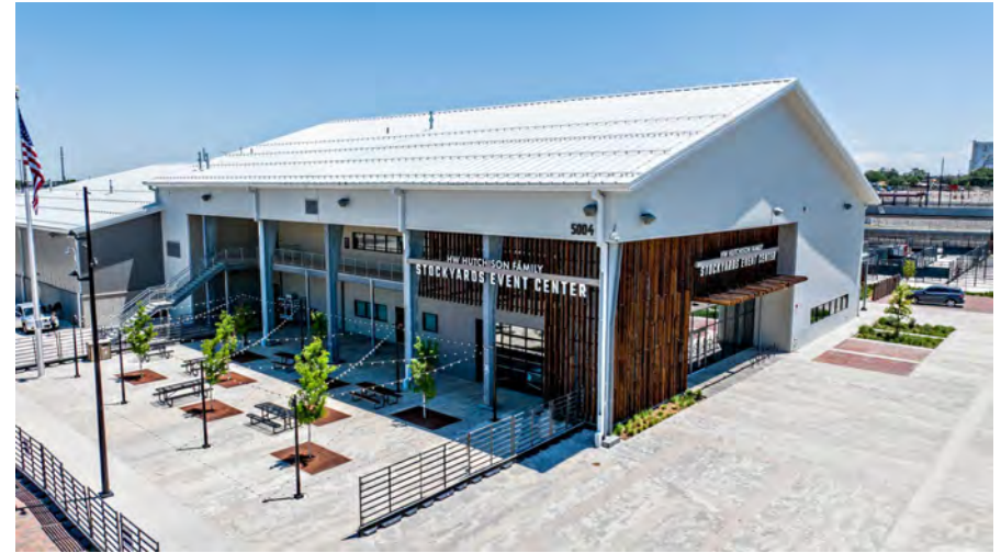
F-7. Stockyards Event Center at National Western Center
