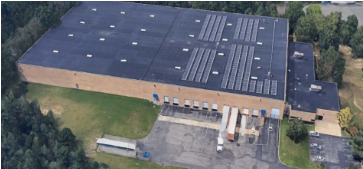
Aerial view of the approximately 430 ft x 240 ft warehouse and attached office. The failed area was located along the east wall.
