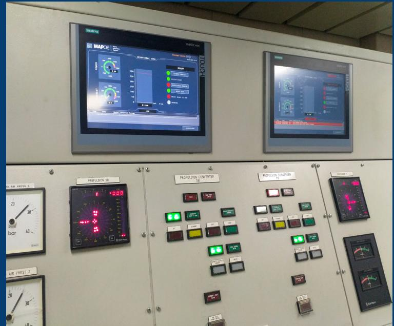
The upgrade delivered enhanced reliability, diagnostics, and ease of maintenance through the integration of modern drives, PLC, and HMI systems. This was achieved with seamless integration with existing ship systems, avoiding major rewiring or infrastructure changes.
