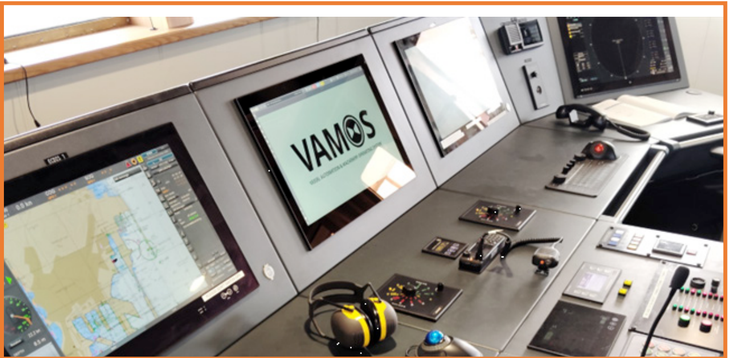
Bridge Console complete with VAMOS 24" Operator Stations.
