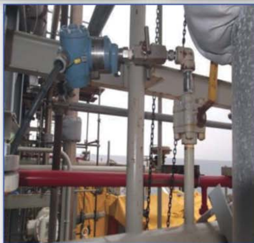
Examples of inadequate supports for piping and instruments
