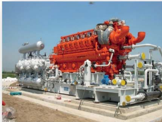
UNDERGROUND STORAGE COMPRESSOR
