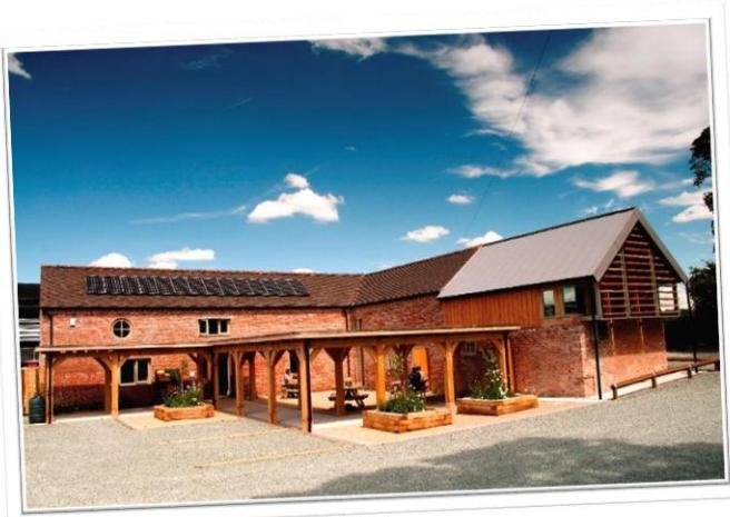
recycled newspaper insulation, sheep's wool insulation, Welsh slate, lime plasters, clay paints and recycled aggregate paving. We also generate our own electricity using PV Panels and generate our own heat using an air source heat pump.
