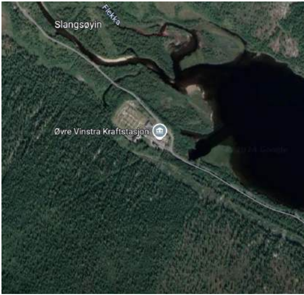
(a) Outlet seen from the Satellite image
