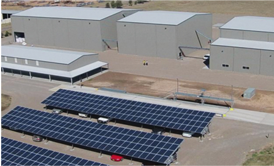
Actual Photo of AOI's Cootamundra, Australia Facility Including its Solar Panels
