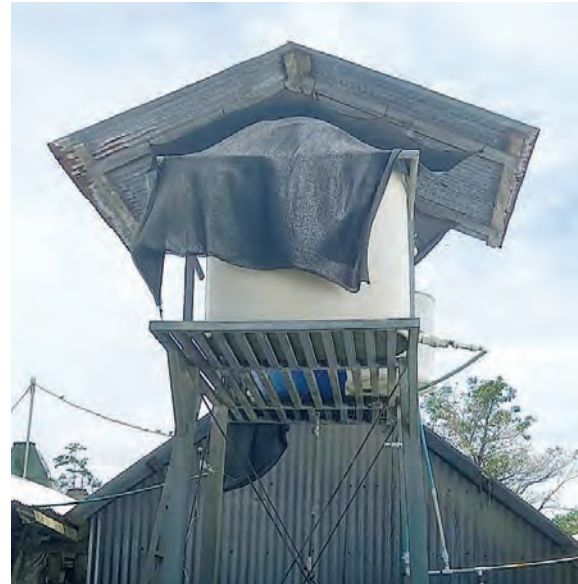
Keeping water cool in elevated white tank with roofing and shade cloth
