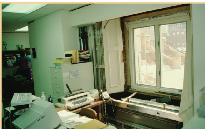
For many years Capitol offices contained a messy assortment of finishes and furniture that didn't date to any one historical period. Note the original woodwork around the modern window, which has been obscured at the top by a modern soffit.
