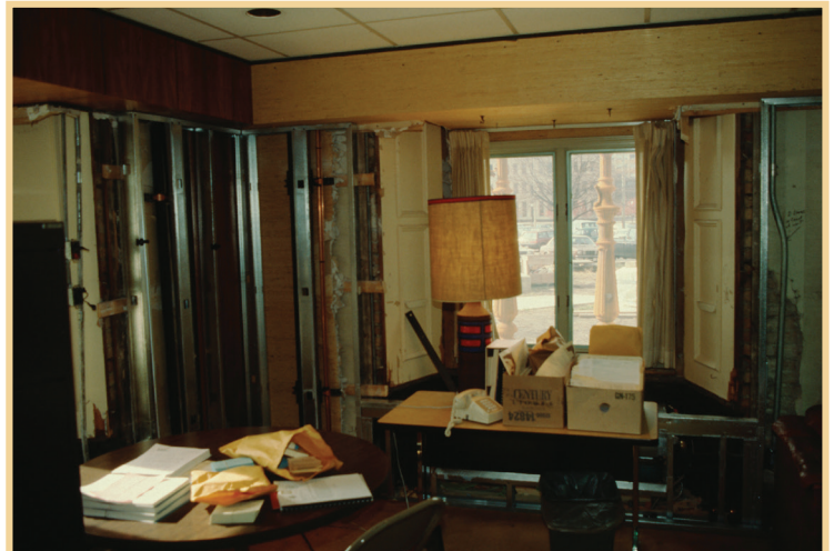
Prior to the restoration, the ground floor offices contained drywall built out from the walls, drop ceilings, fluorescent lights, and modern, inefficient windows.
