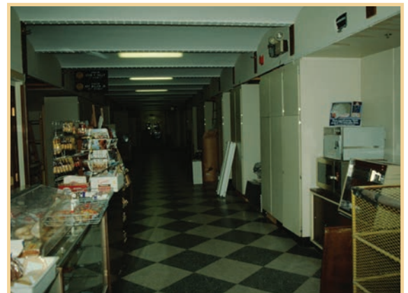
By the late 1980s the Ground Floor corridors were packed with wooden storage cabinets, modern soffits, florescent lights, and, in the south wing, a snack stand.
