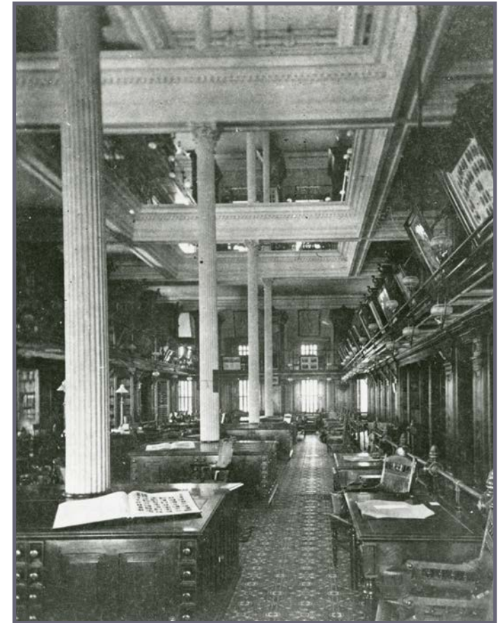
A view of the new State Library from the second floor, circa 1879. Corinthian cast iron columns supported iron beams that ran through the open center of the room at the third and fourth floor levels. These beams supported the weight of the balconies and bookshelves bordering the room on the upper floors.
