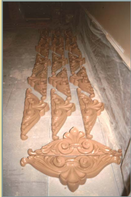
Plasterers cast a large number of decorative elements during the restoration. These pediments were later placed above the doors and carefully woodgrained to have the appearance of walnut.
