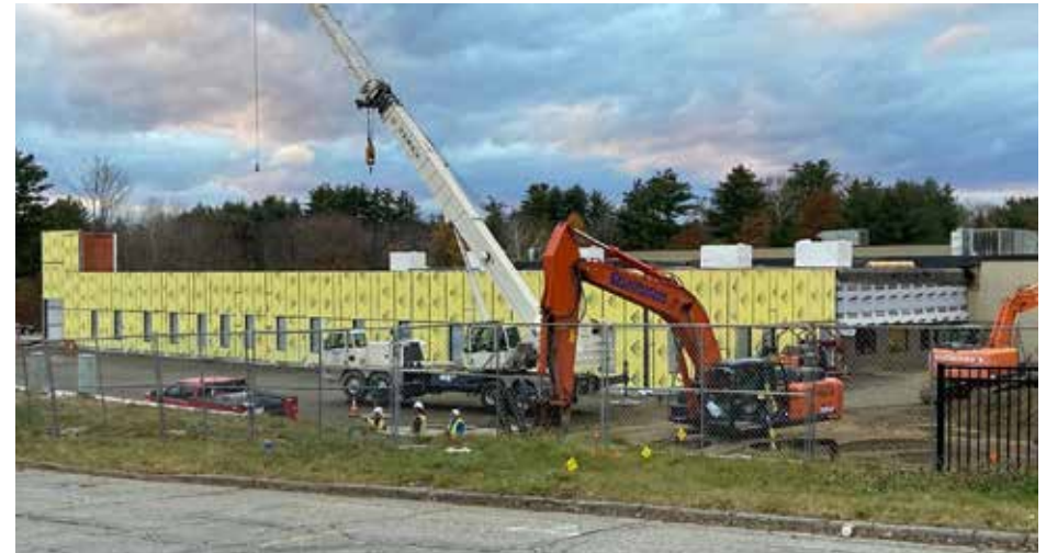
15 Darin Drive production facility during expansion
