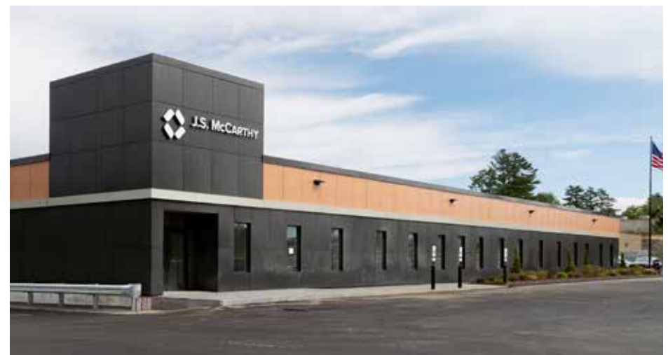
15 Darin Drive production facility after expansion
