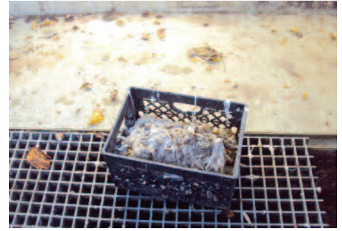
A rigid milk crate filled with rags that were recently raked from the bar screen.
