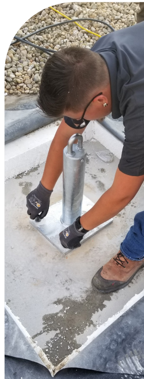
Post Style Roof Anchor
