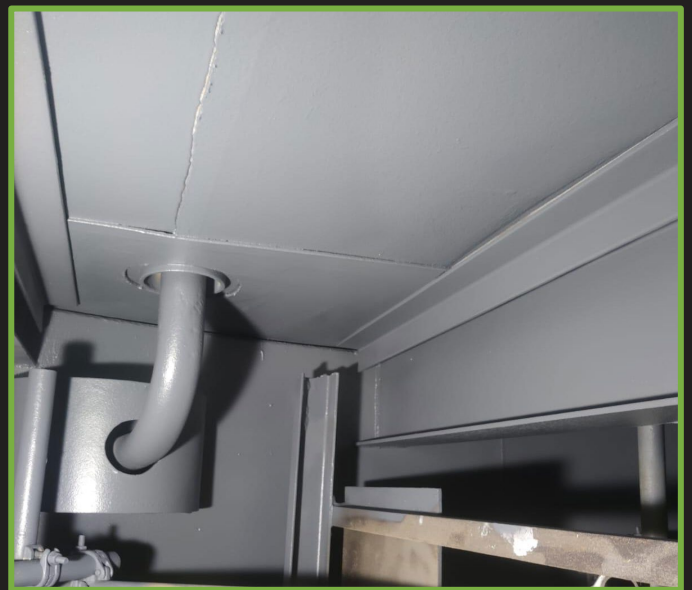
Post lining application of tank roof structure
