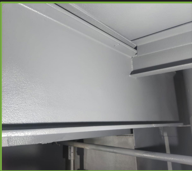
Post lining application of tank roof structure
