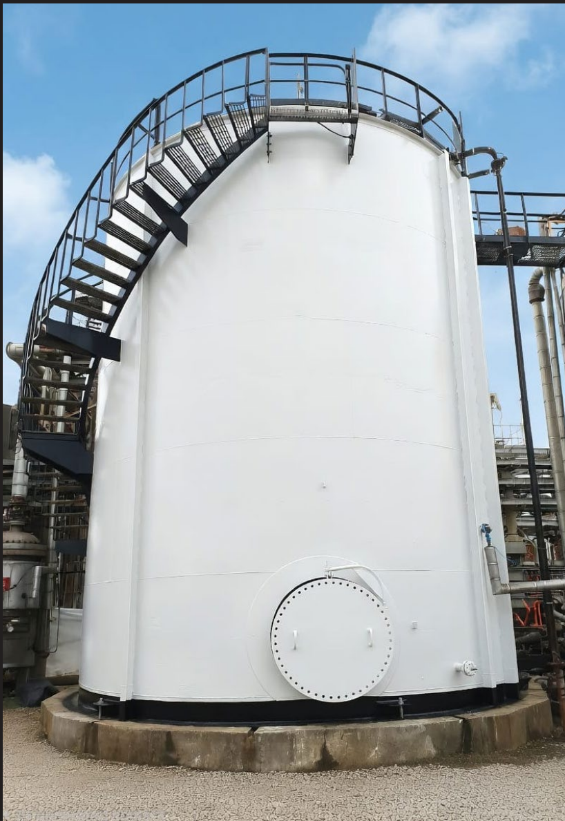
Fully refurbished tank
