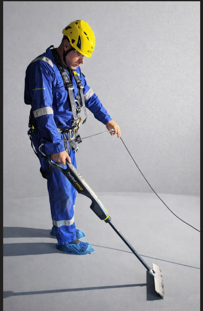
High Voltage Holiday Testing
