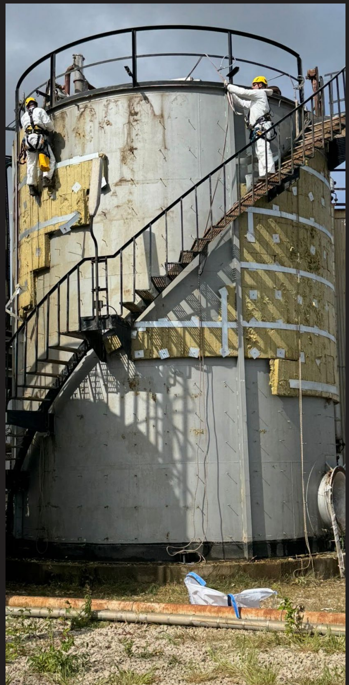
Removing tank insulation using Rope Access
