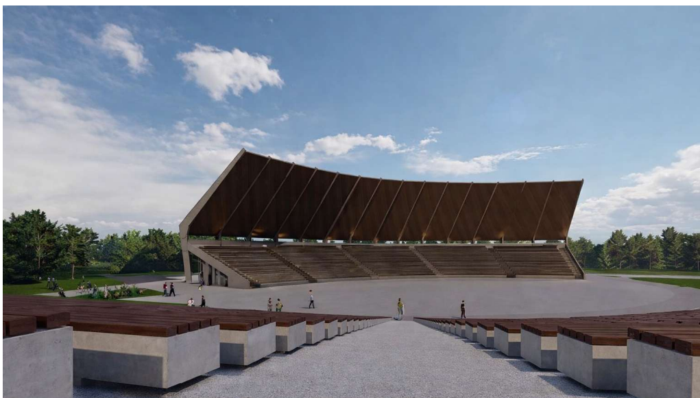
Figure 4: The reconstruction of the Klaipėda Summer Stage
