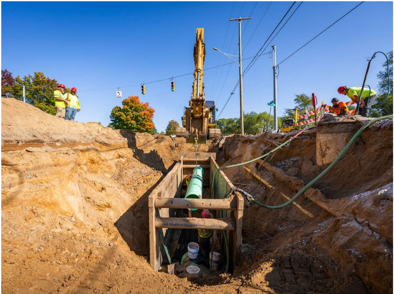
The New Sewer Line
