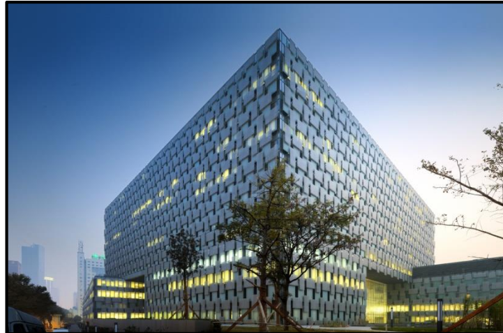
Figura 29- Hospital Nanjing Drum (ARCHDAILY, 2014).
