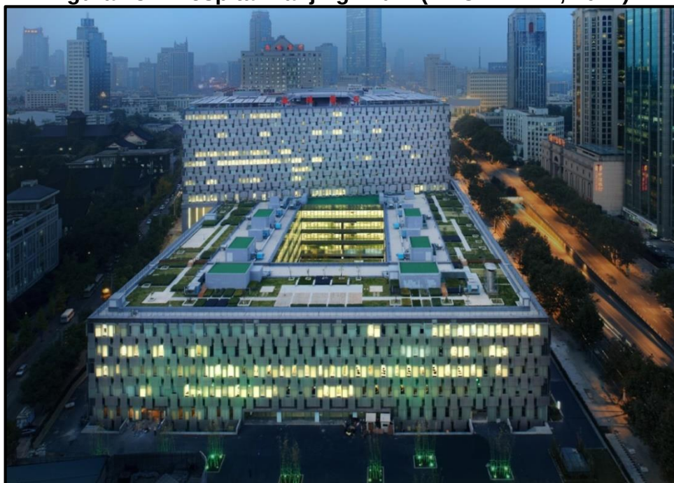
Figura 28 - Hospital Nanjing Drum (ARCHDAILY, 2014).
