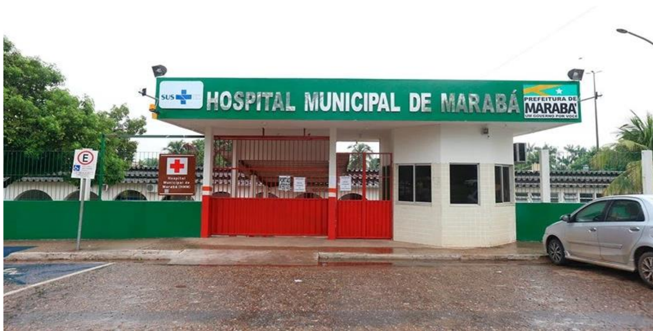
Figura 1 – Vista frontal do Hospital Municipal de Marabá
