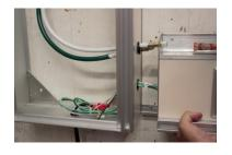
Secure the rail to the building wall/backing material using appropriate hardware [see Step 3 above]
