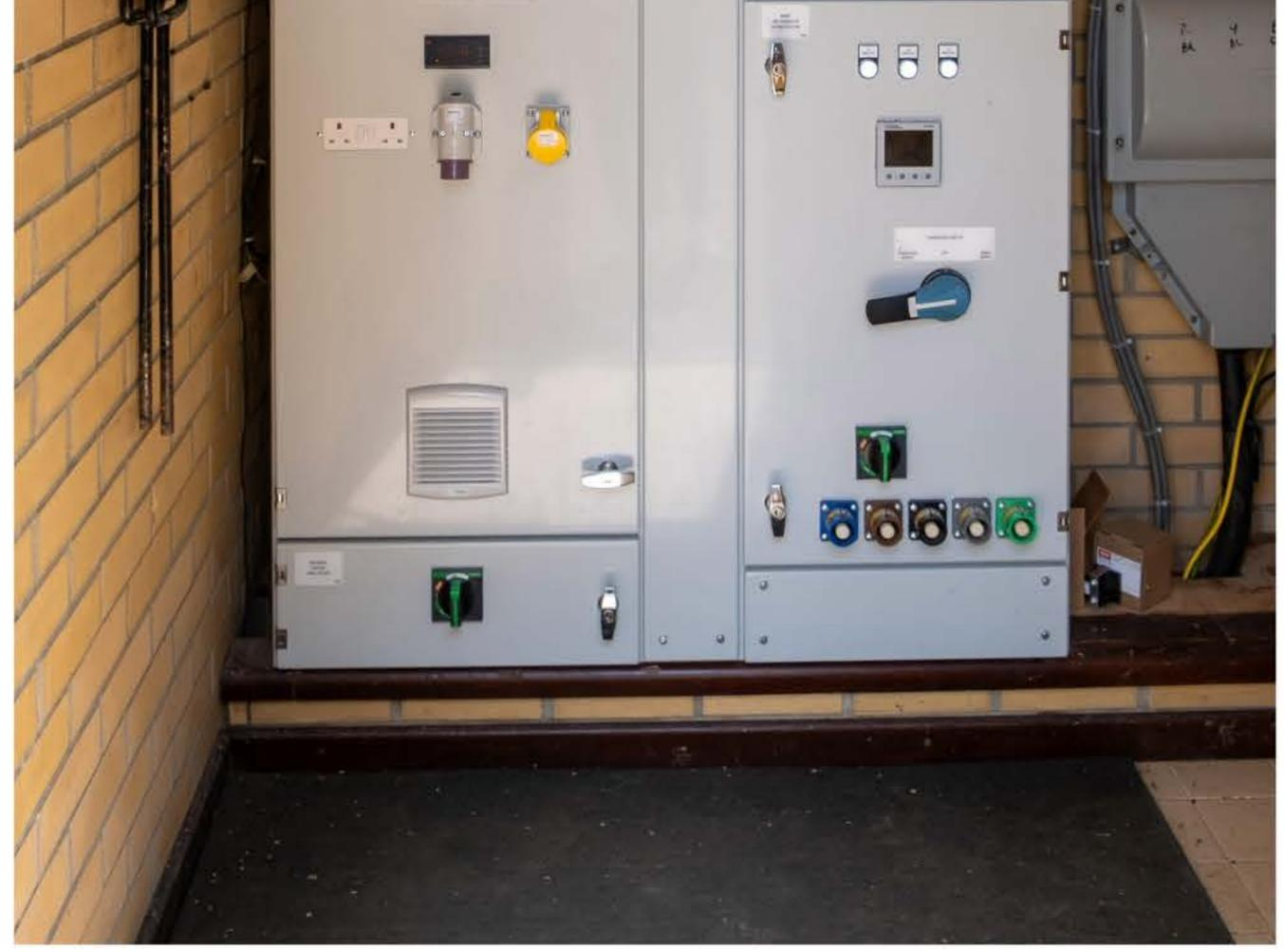
control system was set to incorporate control for a 30kw star/delta pump, power factor correction, control redundancy, PLC and HMI, mobile generator changeover functionality, surge protection and Lee Dickens telemetry integration. Alongside this, the panel would also distribute power to the local feeds such as room heating and cooling, UPS backup and Weed screen panel.
