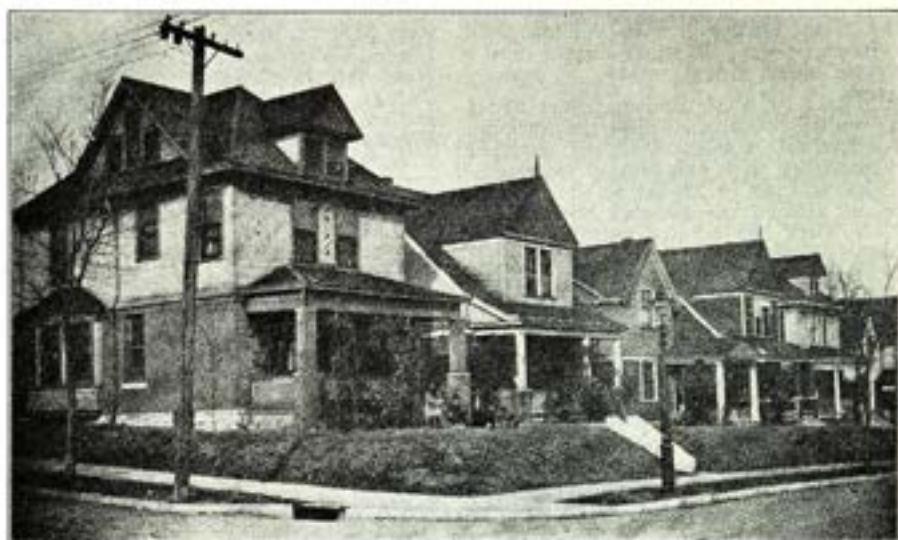
COLORED RESIDENCES—EAST SIDE OF MONTGALL AVENUE
