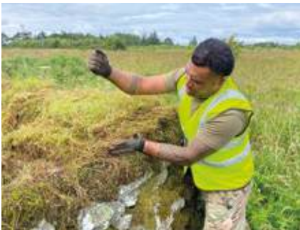
LCpl Bacogacoga soft capping the enclosure
