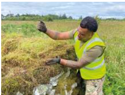
LCpl Bacogacoga soft capping the enclosure
